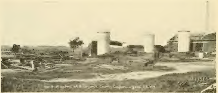
Three Concrete Silos in Perfect Condition After a Wind Storm —Photo by Courtesy of Sanders Pub. Co., Chicago
